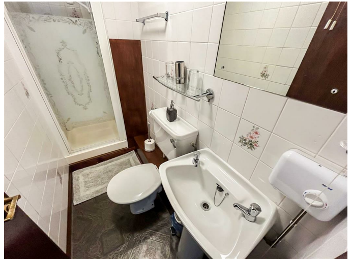
Having hand wash basin, W/C and shower cubicle with wall mounted shower.
