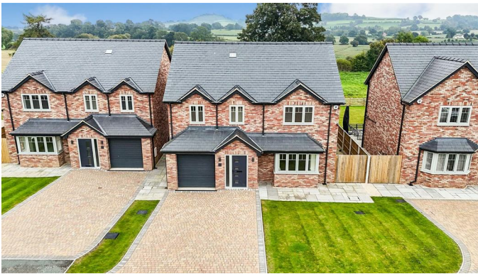
To The Front Of The Property
