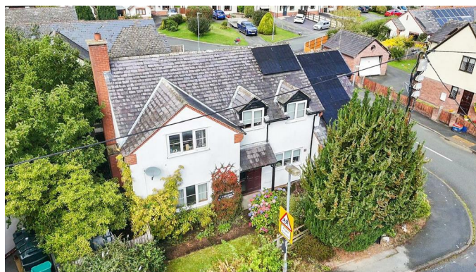
To the Front of the Property
